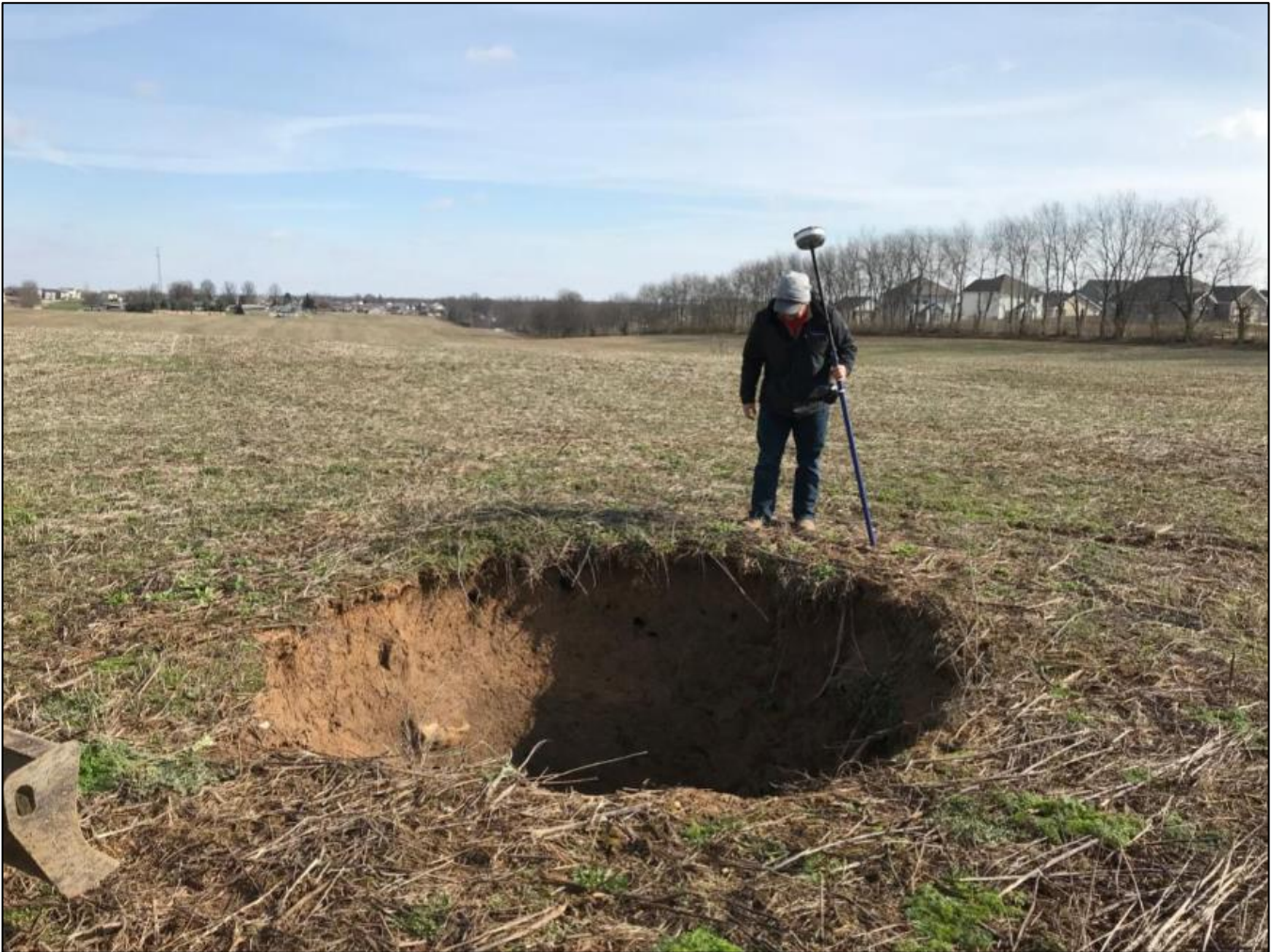
Figure 107: Sinkhole in Scott County (Image)
