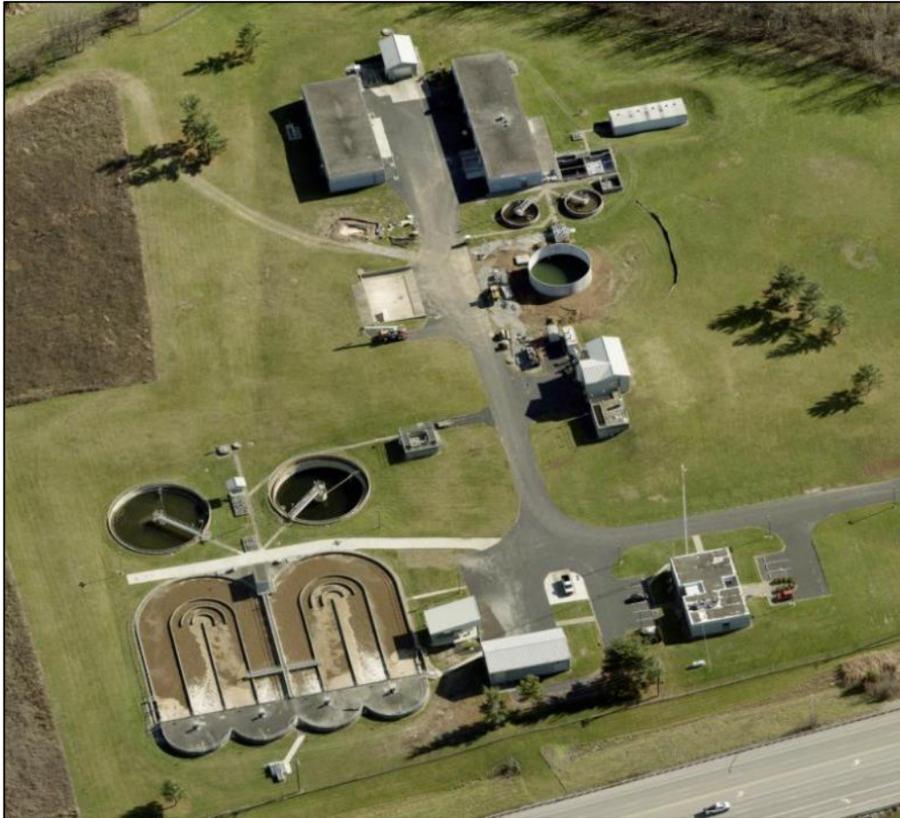
Figure 51: Aerial Imagery of Wastewater Treatment Plant #2 (Image)
