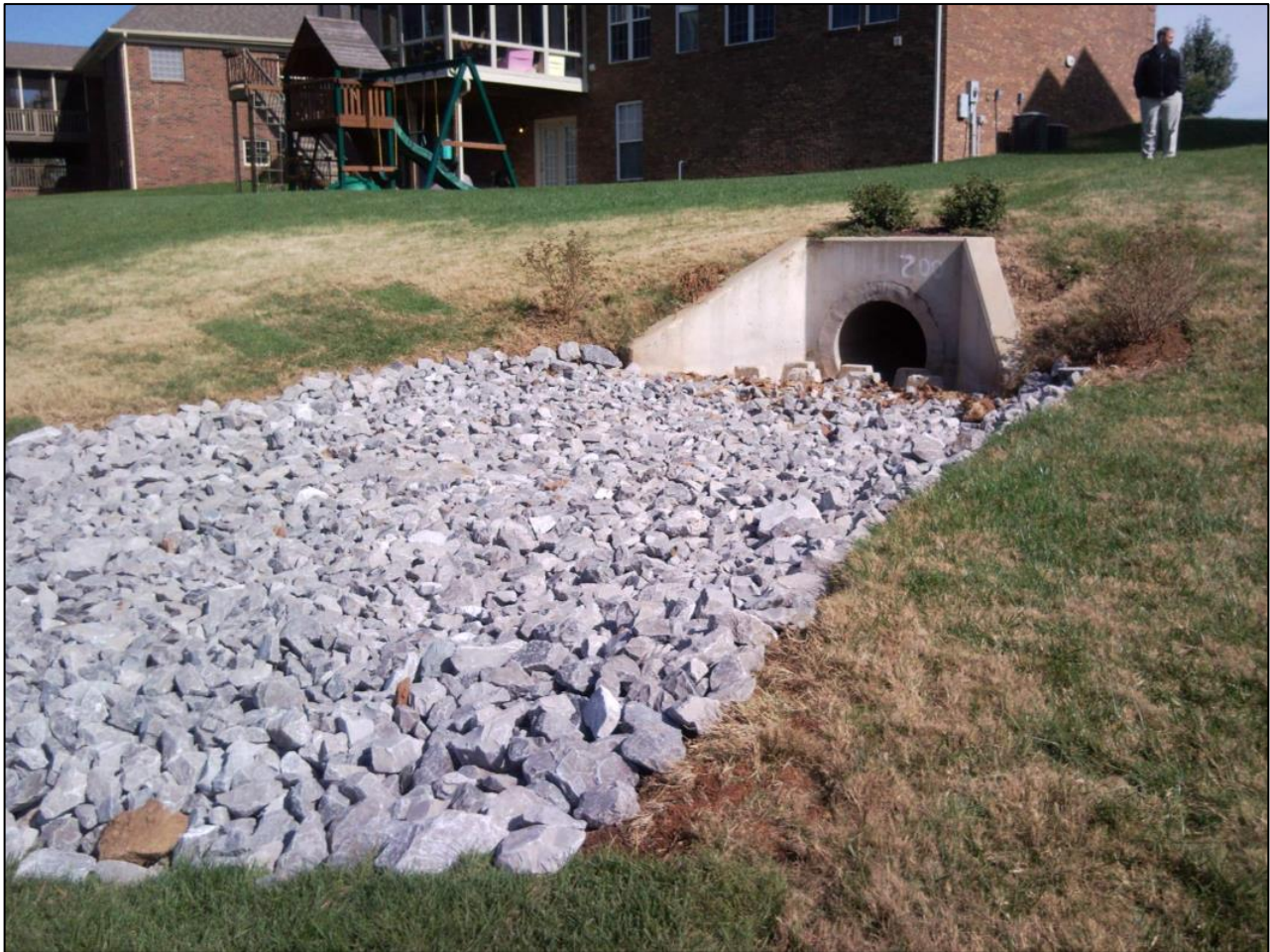
Figure 44: Storm sewer Outfall (Image)
