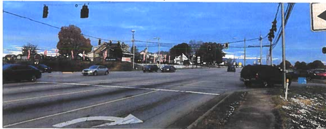
Intersection of US 25 and US 62 Bypass
